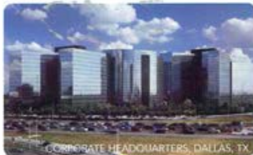
CORPORATE HEADQUARTERS, DALLAS, TX
